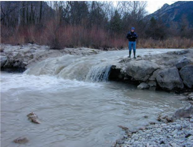
**Fig. 9** Photographs showing destabilization of infrastructures within the Drôme catchment (France) because of channel degradation. (A) Bridge at Die destabilized during the November 2003 flood. (© F.Liébault.) (B) Undermined weir at Luc-en-Diois requiring restoration.
