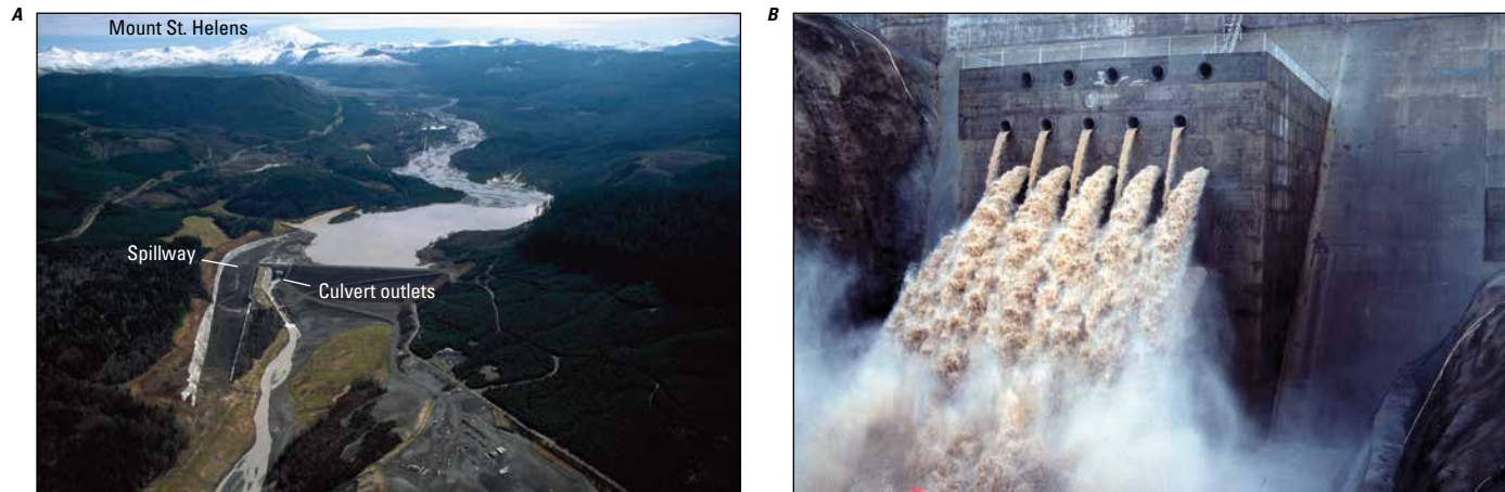
Figure 8. Views of sediment retention structure on North Fork Toutle River looking upstream. A , Oblique aerial view. B , Water passing through rows of culverts embedded in face of structure (see A for location). U.S. Army Corps of Engineers photographs from approximately 1990.
