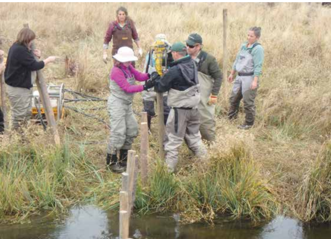
A work party builds a beaver dam analog in Bridge Creek, Oregon, a tributary of the John Day River. Beaver-related restoration tactics are being used to restore riparian areas, expand wildlife habitat, and improve forage for livestock. USDA Forest Service photo.
