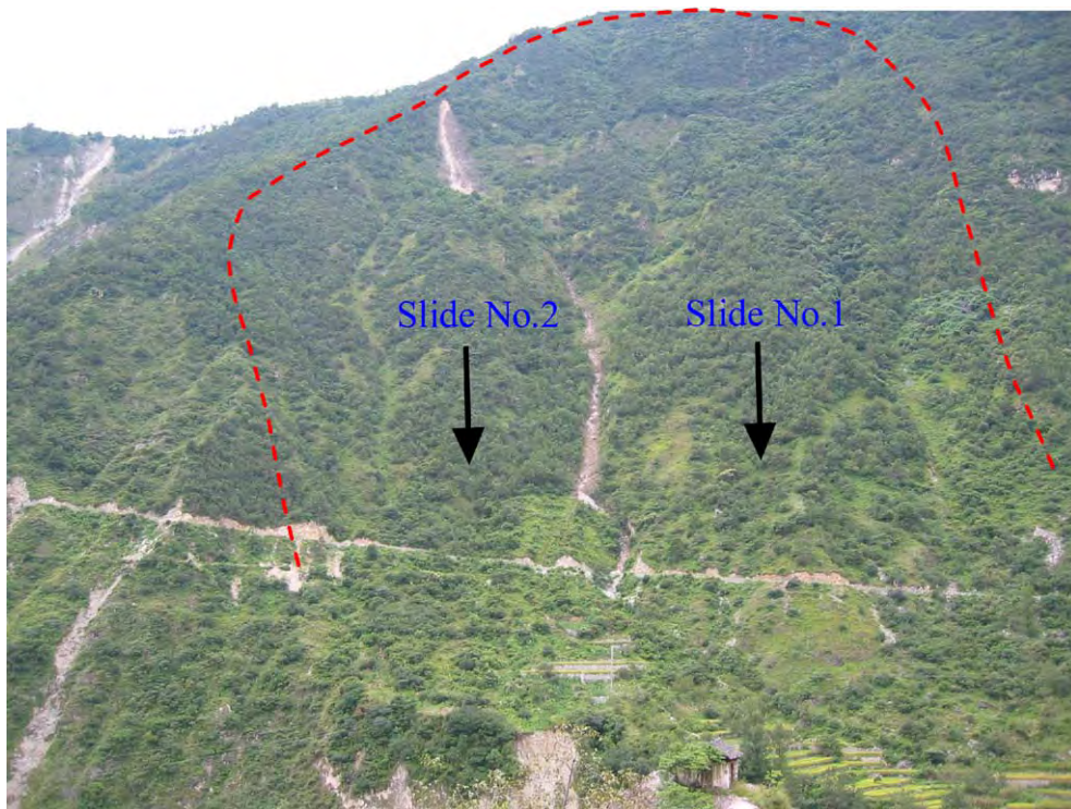
Fig. 6. Photograph showing the landslide site (view is to the west). The failure main scarp is marked with a dashed line, and the location of the site is shown in Fig. 4.
