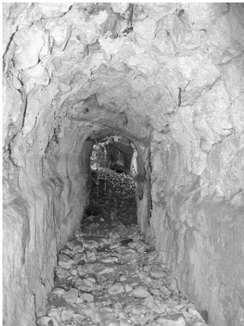
Fig. 22. Roman aqueduct. View of one tract of the tunnel that we discovered between Santa Maria Oliveto and Pozzilli. Note the ancient water level, indicated by the top of the travertine growth over the walls. Dimensions are 1.6 m (height) and 0.6 m (width). The right side and the bottom are here directly excavated in the carbonate rocks, whereas the left side and the round-arch are built with stone masonry.
