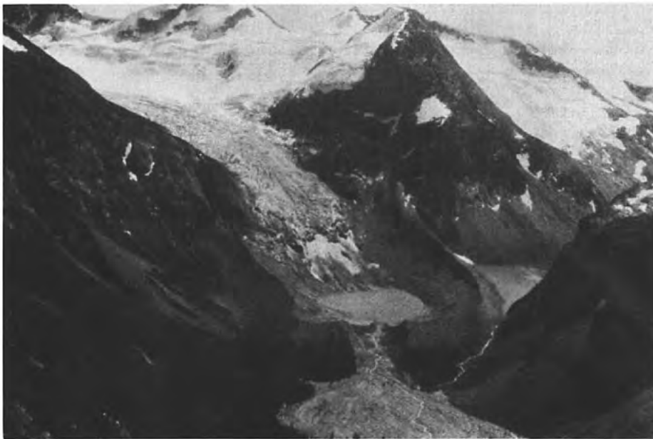
Figure 10B. Photograph of Nostetuko Lake and Cumberland Glacier, British Columbia, Canada, in August 1983, after failure of the moraine dam. Cross section of dam shown in Figure 13. (Photograph by Michael Church, University of British Columbia.)
