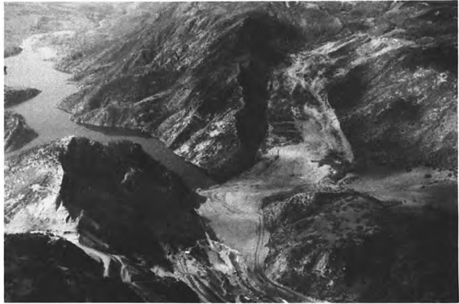
Figure 11. Photograph of the 1983 Thistle, Utah, landslide (right) and its temporary impoundment, Thistle Lake (left), in September 1983. The lake inundated the town of Thistle and was then drained late in 1983 by a bedrock tunnel constructed through the mountain at lower left.
