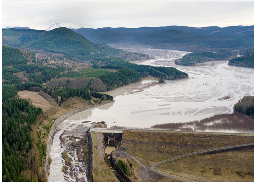
Figure 3. Sediment Retention Structure (SRS) and sediment plain in winter 2012–2013 (following implementation of the first spillway raise, in summer, 2012) (courtesy of USGS Cascades Volcano Observatory). [Colour figure can be viewed at wileyonlinelibrary.com ]
