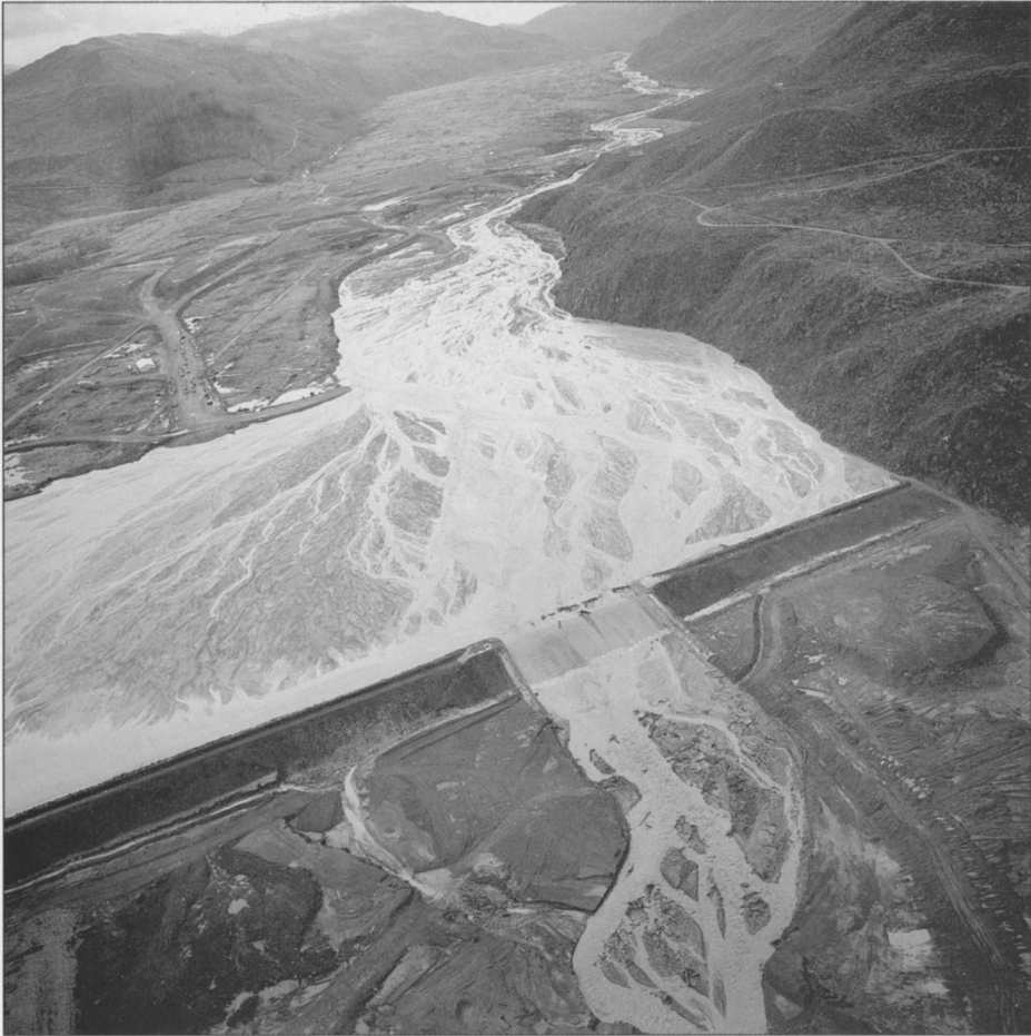
A freshet temporarily breached the spillway on the North Fork Toutle River debris retention dam in December 1980. The Corps repaired the breach and subsequently strengthened the structure.
