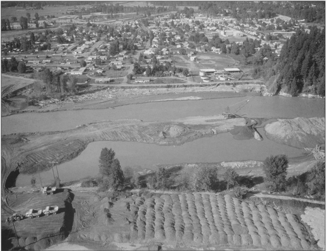
An example of dragline dredging on the Toutle River. Dredged material has been deposited in mounds or rows in a disposal area in the foreground of the photograph.
